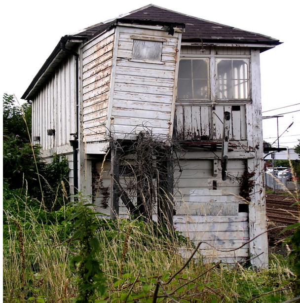
Signal Box Before Renovation
