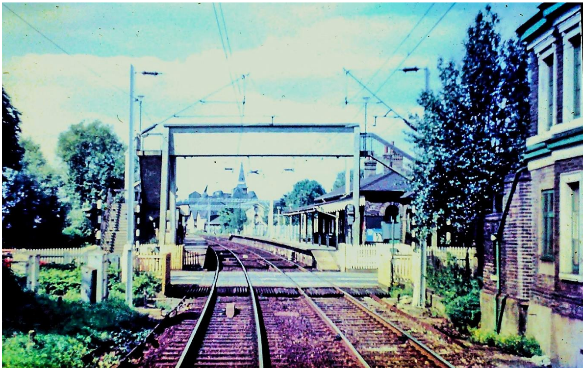
The above picture was taken in August 1971 from the driving cab of an electric multiple unit train as it approached St Margarets station from Rye House. The old hand wound gates had been replaced by the modern lifting barrier type in November 1970. To the right can be seen part of the original 1843 station building, used after the last Stationmaster had left until the early 1970s as a railway workers rented home. Very prominent in the picture is the concrete footbridge erected in 1958/9 as part of the electrification of the line. Electric trains, after testing trials during the early part of the year, took over the passenger services in November 1960.
